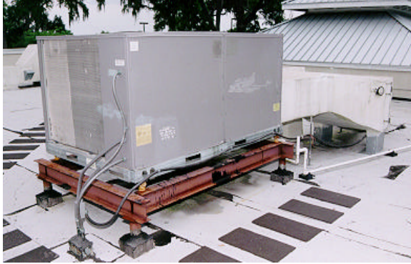
Rooftop unit with ducted supply and return
