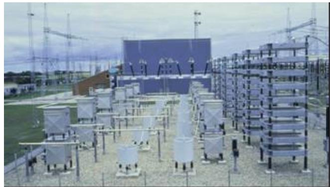
Fig. 1. HVDC converter station with AC filters in the foreground and valve hall in the background
