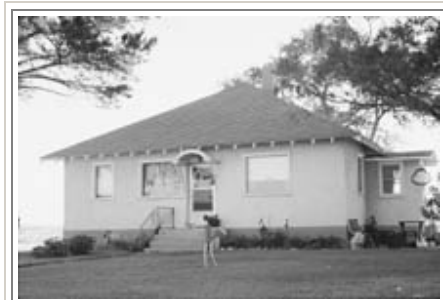
The Scott house was built outside of Gordon, Nebraska, in 1936. It is a classic "Nebraska style," or load-bearing straw-bale house, in that the bale walls carry the roof and lateral loads.
