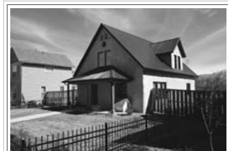
Post-and-beam straw-bale house built in Colorado Springs, Colorado. It is actually two stories in the back, because the lot slopes steeply.
