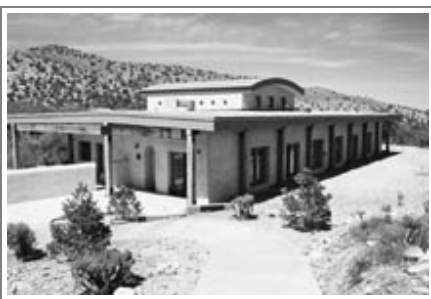
Large post-and-beam straw-bale house outside Moab, Utah. The nearly 100-year-old timbers used in this house were salvaged from a railroad trestle that once crossed the Great Salt Lake.
