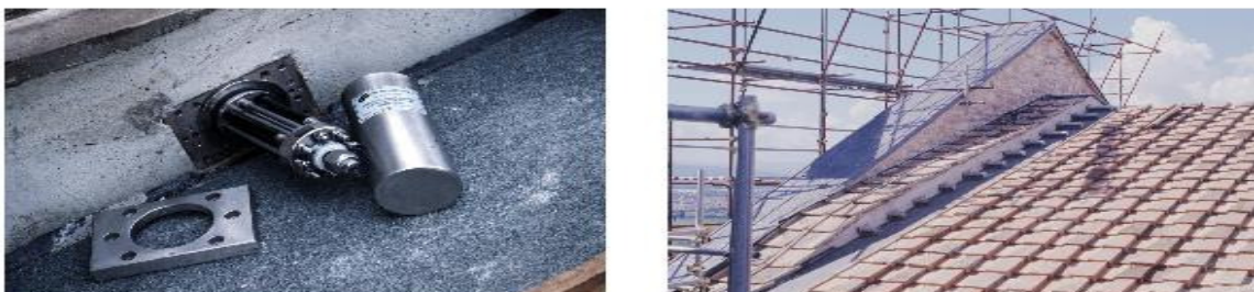
Figure 3 SMA Devices in the Basilica of St Francesco of Assisi [Castellano et al., 2000].
