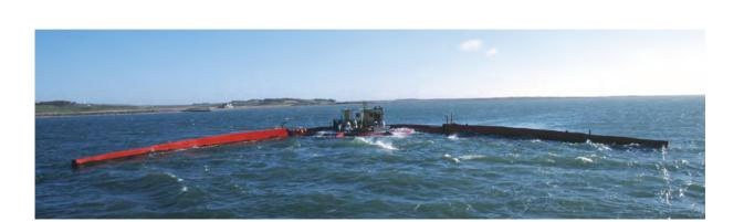
The Wave Dragon is an overtopping device, that combines a double-curved overtopping ramp and two reflector wings, which focus energy towards the ramp. The waves surge up the ramp, as if it were a beach, and behind the ramp a reservoir collects the overtopping water. Multiple variable-speed propeller turbines are used to convert this low-pressure head into electricity using standard type AC generators. The device is slack-moored and is able to swivel in order to always face the wave direction.
