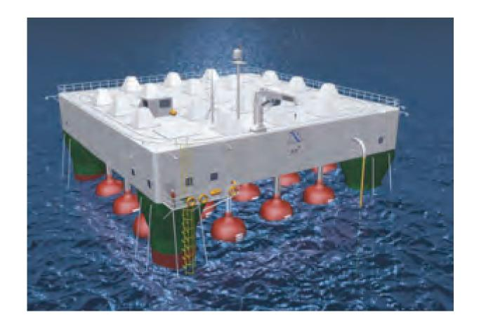
The Buldra platform uses "eggs" mounted below the platform to capture wave energy. As waves pass below the platform the "eggs" rise and fall with each wave. This mechanical energy is then converted into electricity on the platform. The platform itself floats, which allows it to be stationed in any water depth. Power generated on the platform is brought to shore via cable.
