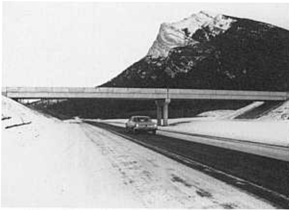
Three Sisters Overpass, Alberta, Canada.
