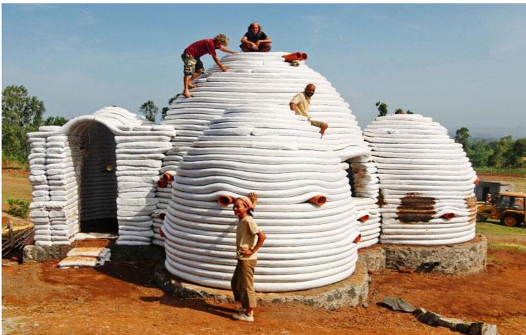
**Figure 2:** A typical superadobe structure
