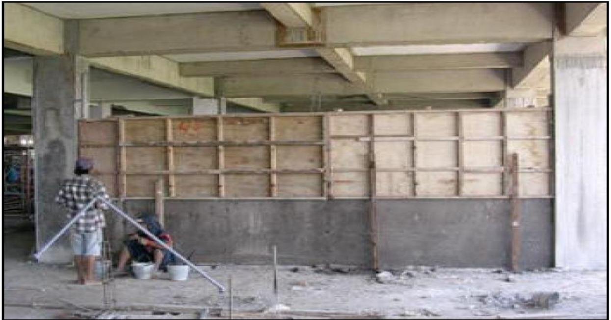
Figure 1.3 Cast in-situ LFC wall in Surabaya, Indonesia.
