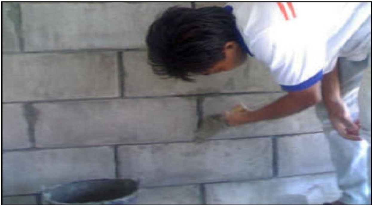
Figure 1.1 LFC blocks being used in a housing project in Malaysia.
