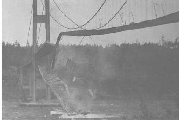
Figure 4.7: Failure of the Tacoma Bridge
