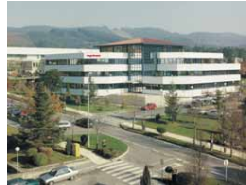
The Ingeteam Head-Office at the Zamudio Technology Park.
