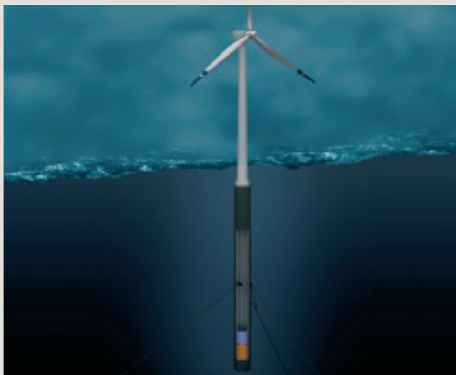
The wind turbine is mounted to a 120 m high floating concrete substructure.
