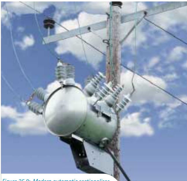
Figure 25.8: Modern automatic sectionaliser
