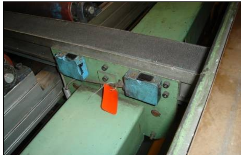
Photo cells damaged - replaced
