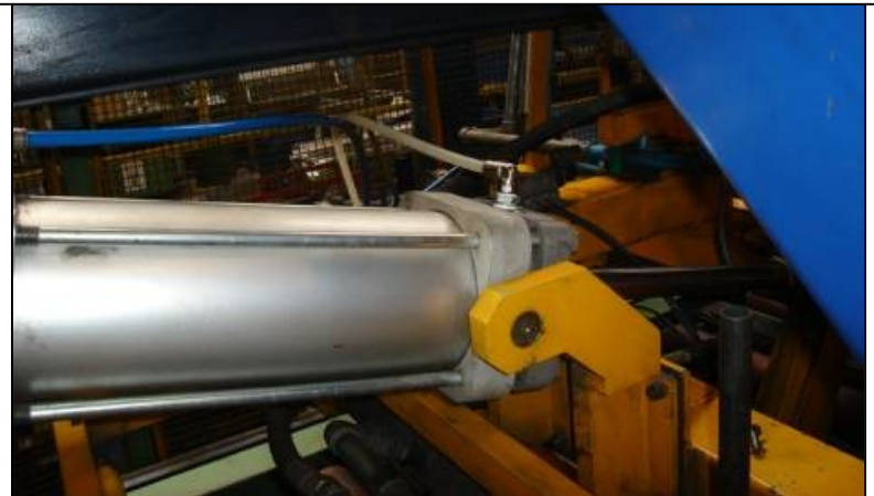
New pipe and fitting to cylinder
